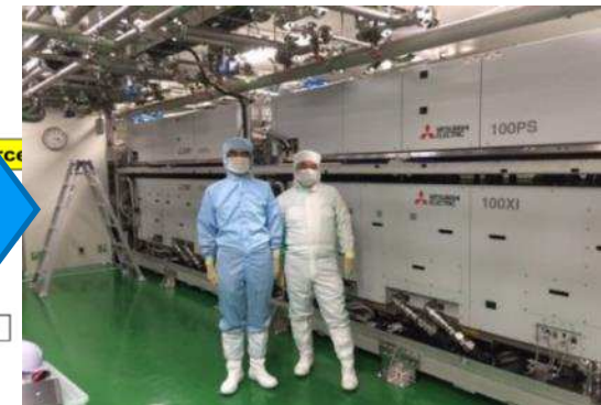
Amplifier system installation in 2016
